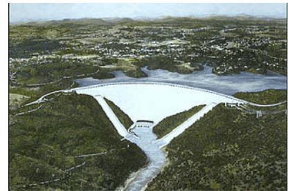
An artist's rendering shows a 1978 design for the Auburn dam that would have been 685 feet high and store 2.5 million acre feet of water.
