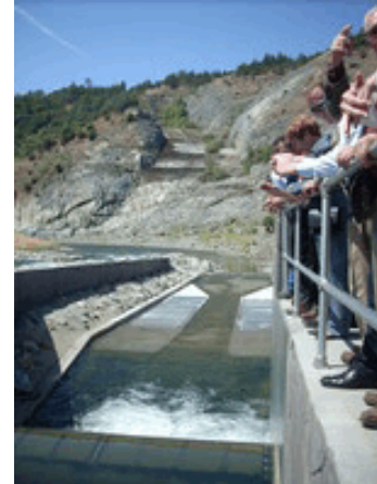
Members of the crowd at Thursday's dedication of the American River pump station project watch as water flows are increased into a man-made section that includes underwater filters that collect water for the pumps
