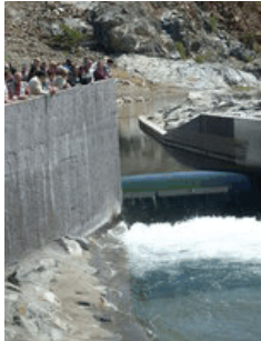
Members of the crowd at Thursday's dedication of the American River pump station project watch as water flows are increased into a man-made section that includes underwater filters that collect water for the pumps
