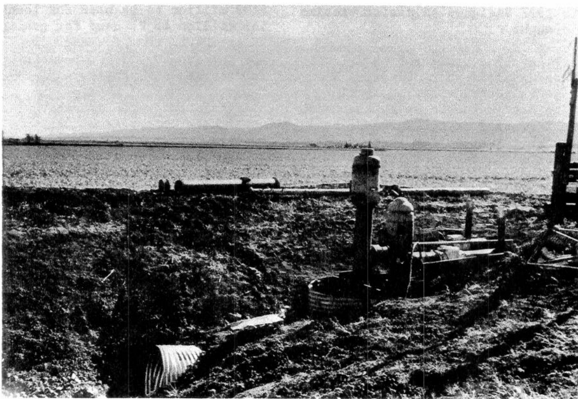
35. Drought aid to farmers. During the drought, several programs were made available to implement soil and water conservation practices. The photographs show a newly lined ditch (to prevent seepage loss) and a tailwater return system. (Soil Conservation Service photos.)
