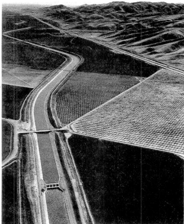
53. The manmade river. The California Aqueduct, shown here meandering through the San Joaquin Valley, saw substantial reductions in the amount of water transported in 1977, but will deliver all water needed in 1978.
