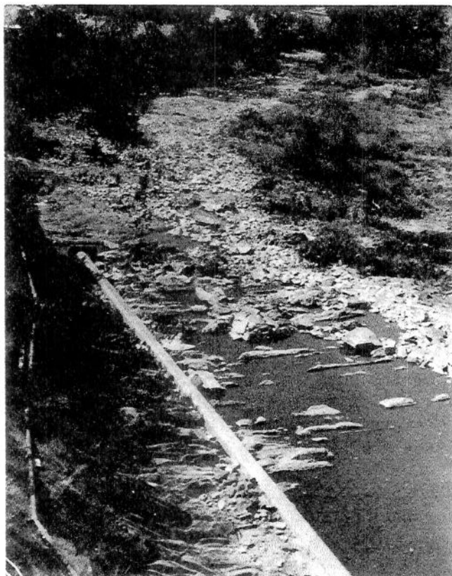
18. Little help for the valley farmer. This photograph, taken below Stony Gorge Reservoir, shows Stony Creek on August 31, 1977. Storage upstream in both Stony Gorge and East Park Reservoirs, serving the Orland Water Users Association, was depleted early in 1977.
