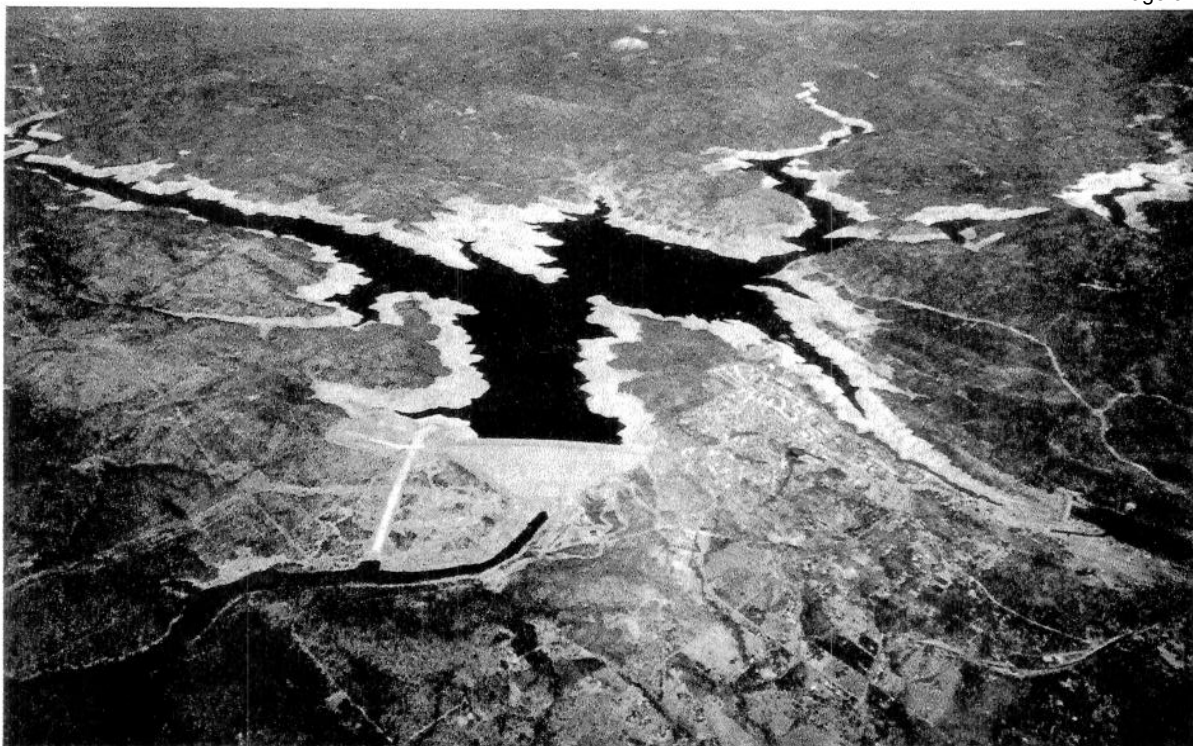
7. Low on reserves. Lake Oroville as it appeared on September 30, 1977. Storage on that date was only 1 100 cubic hectometres (915,000 acre-feet), or about one-fourth of capacity. Lake Oroville reached its lowest point on September 7.
