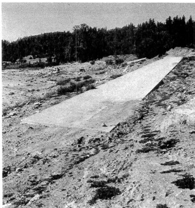
24. Where can I launch? The question was asked often in 1977 as reservoirs receded to record lows. This boat ramp at Rollins Reservoir in Nevada County was left high and dry. When this photograph was taken, the water level was another 30 metres (100 feet) down the slope.
