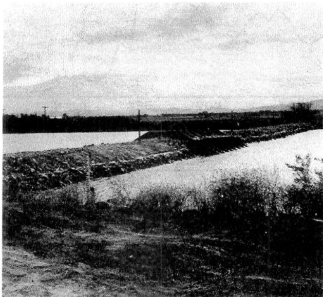
6. Guardian of the South Delta. The Dutch Slough barrier, west of Antioch, prevented the inflow of salt water and kept the salt content at an acceptable level.
