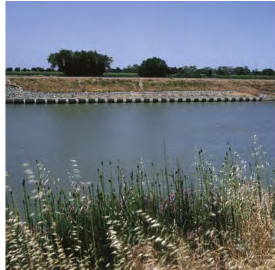
Experimental levee maintenance programs are being conducted at various locations in the Delta to determine better ways to protect the environment while maintaining flood control. This photo shows a project to develop a berm that will provide for environmentally important shaded aquatic habitat.
