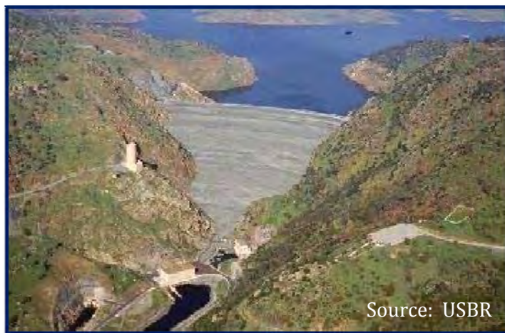
Figure 1-1. New Melones Dam
