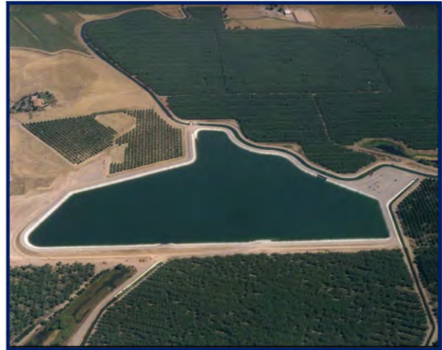
Figure 3-4. North Side Regulating Reservoir
