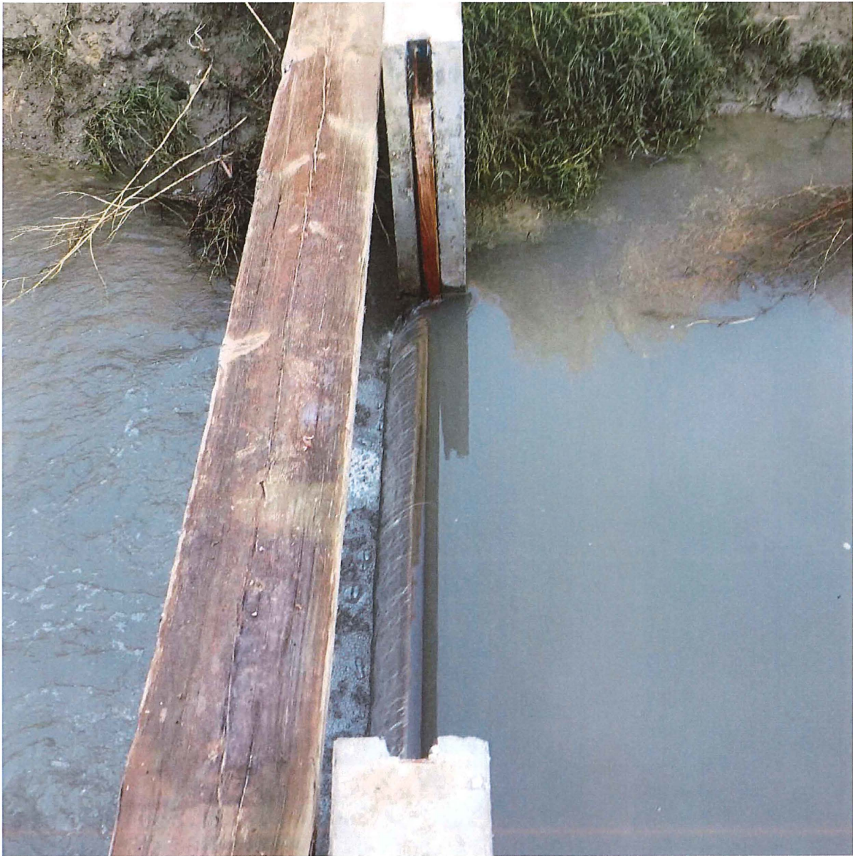
Photo of Bethany Drain weir by Rick Martinez, November 30, 2015.
