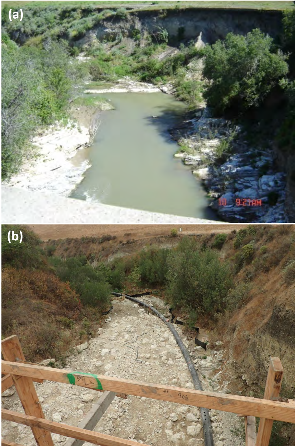
Figure 63: Photo point (T-39) collected at Salsipuedes Creek at Hwy 1 Bridge in May 2005 and (b) September 2020 (during Caltrans bridge replacement project).
