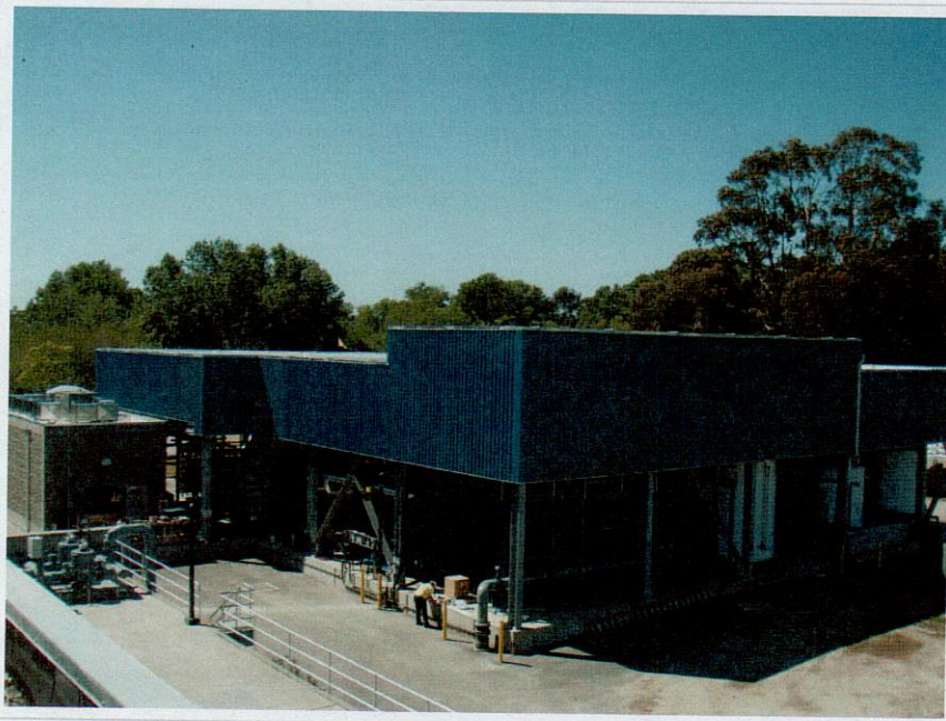
Completed project with fully functional equipment
