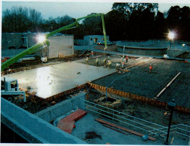
Pouring the foundation for the new treatment facility
