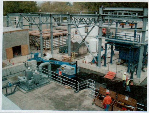
MF/RO equipment being installed
