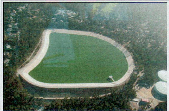
Rehabilitated in 2006 for recycled water storage
