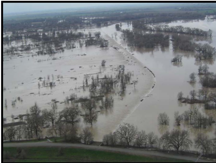
Fremont Weir and Sacramento River Looking North on February 20, 2004
