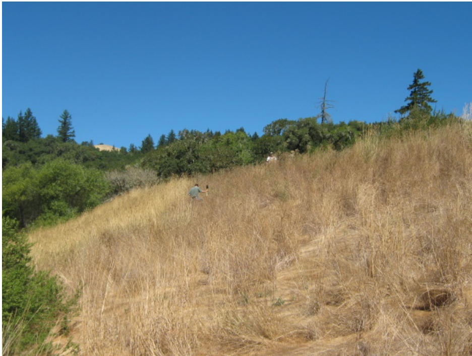
RESERVOIR #1 DAM LOOKING NORTHEAST
