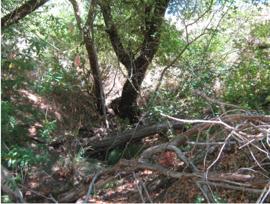
DOWNSTREAM CHANNEL LOOKING BACK TOWARDS RESERVOIR #1 DAM
