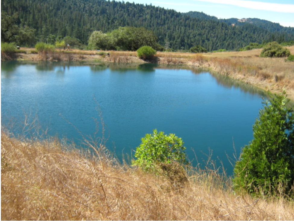
RESERVOIR #2 LOOKING WEST
