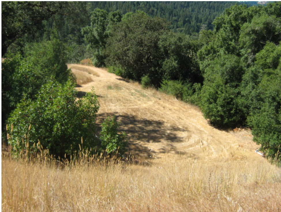
ATOP RESERVOIR #2 DAM LOOKING WEST
