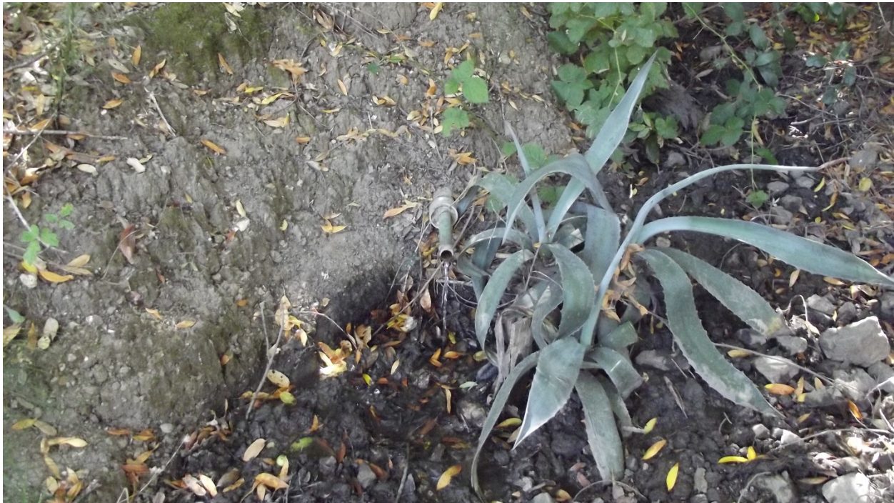
Figure 6: Horizontal pipe emerging from the bank of the stream connecting the reservoirs
