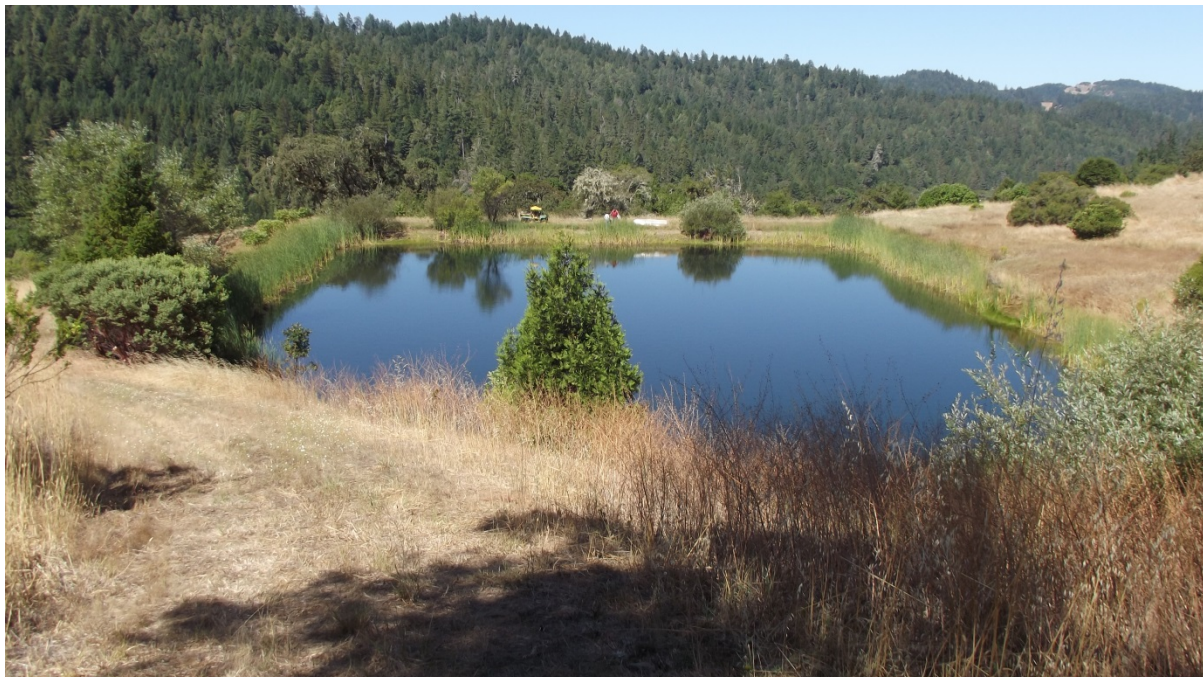
Figure 3: Reservoir 1 facing downstream to the west. The dam can be seen on the far side of the reservoir.
