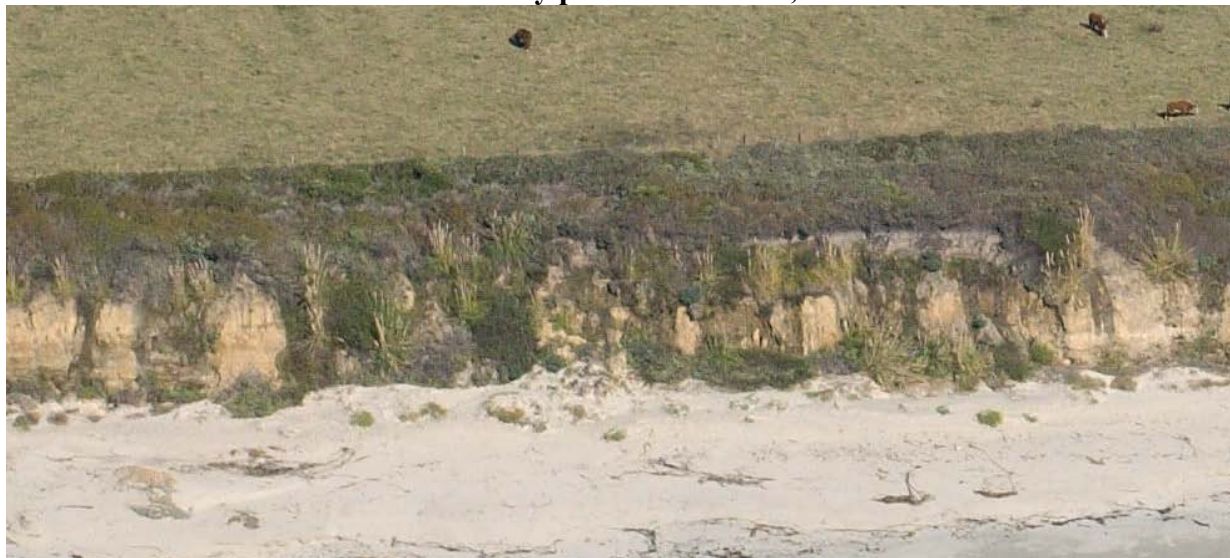
Figure 15: Close up of seepage and pampas grass on cliff between Hanson's bluff survey points #3 and #4, October 2005.
