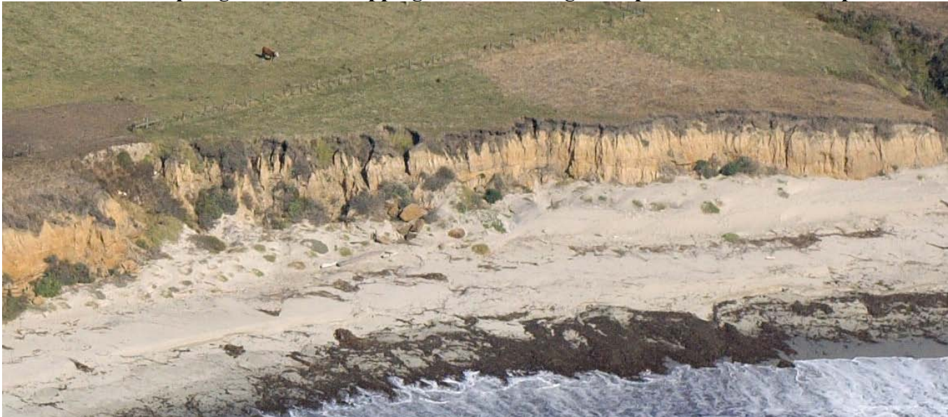
Figure 9: Cliffs at El Sur Ranch Pasture 7 – October 2005 Close up of groundwater sapping erosion causing scalloped erosion head scarps
