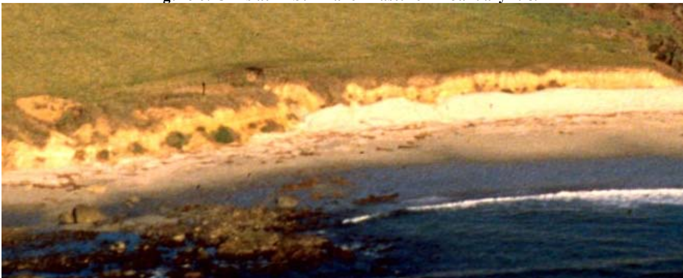
Figure 6: Cliffs at El Sur Ranch Pasture 7 – January 1989
