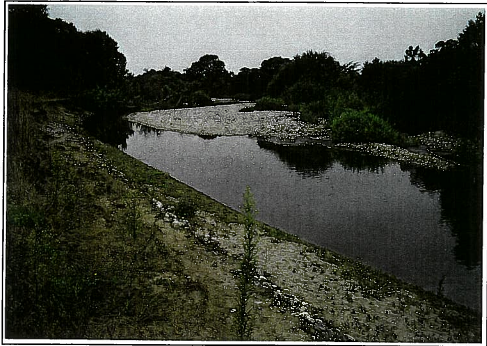
Plate 9. View upstream of the Big Sur River about 1,600 feet downstream of the right bank tributary. The bank attached bar on the left bank is causing erosion and retreat of the right bank. Note the colonization of the gravel bar by willows and alders.
