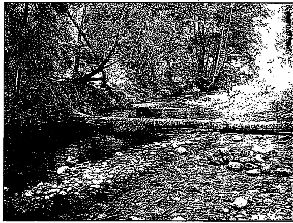
LWD related scour pool. (PBSRM 0.50)
