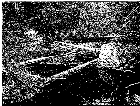
Old diversion dam site. (PBSRM 0.13) This existing structural grade control feature is one of 8 old instream grade controls that affect channel width/depth dimensions in PBS.
