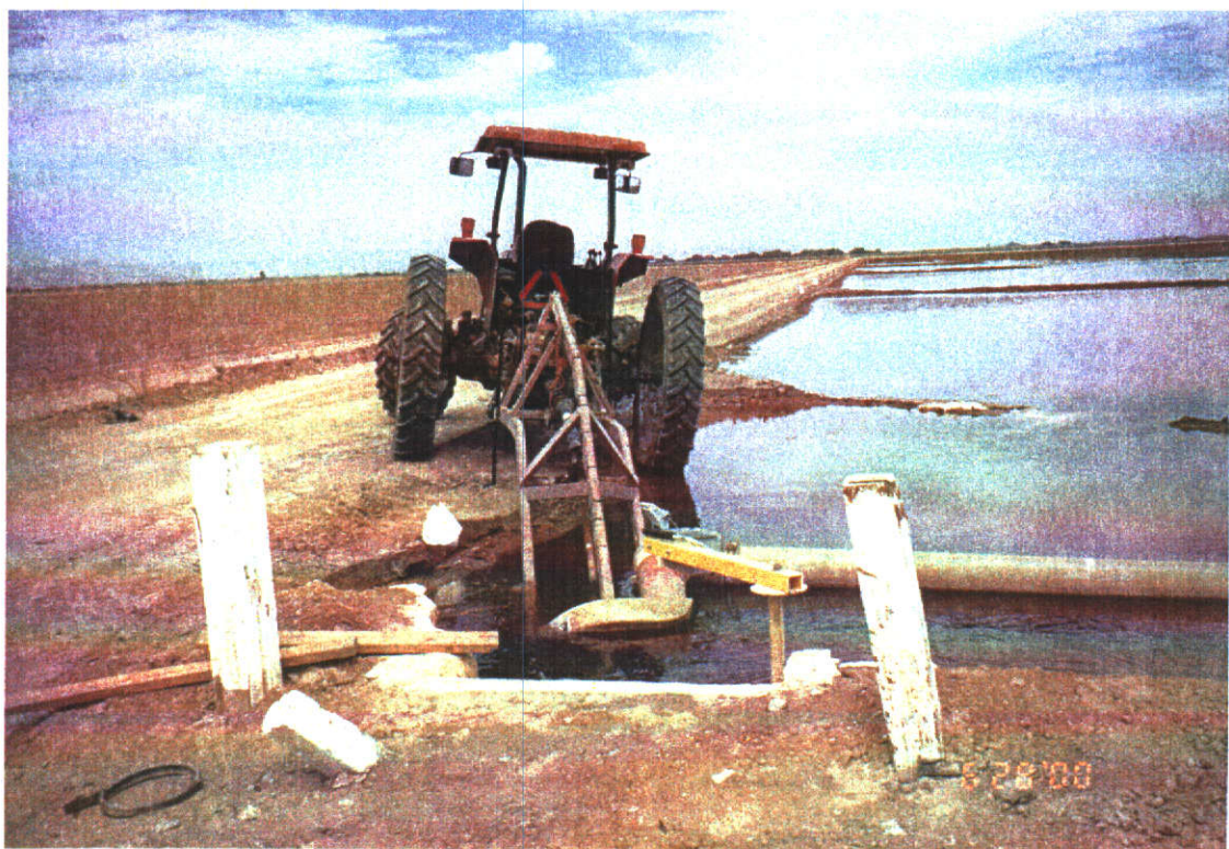
No. 10 Portable tail water pump back system used during a leaching irrigation.
