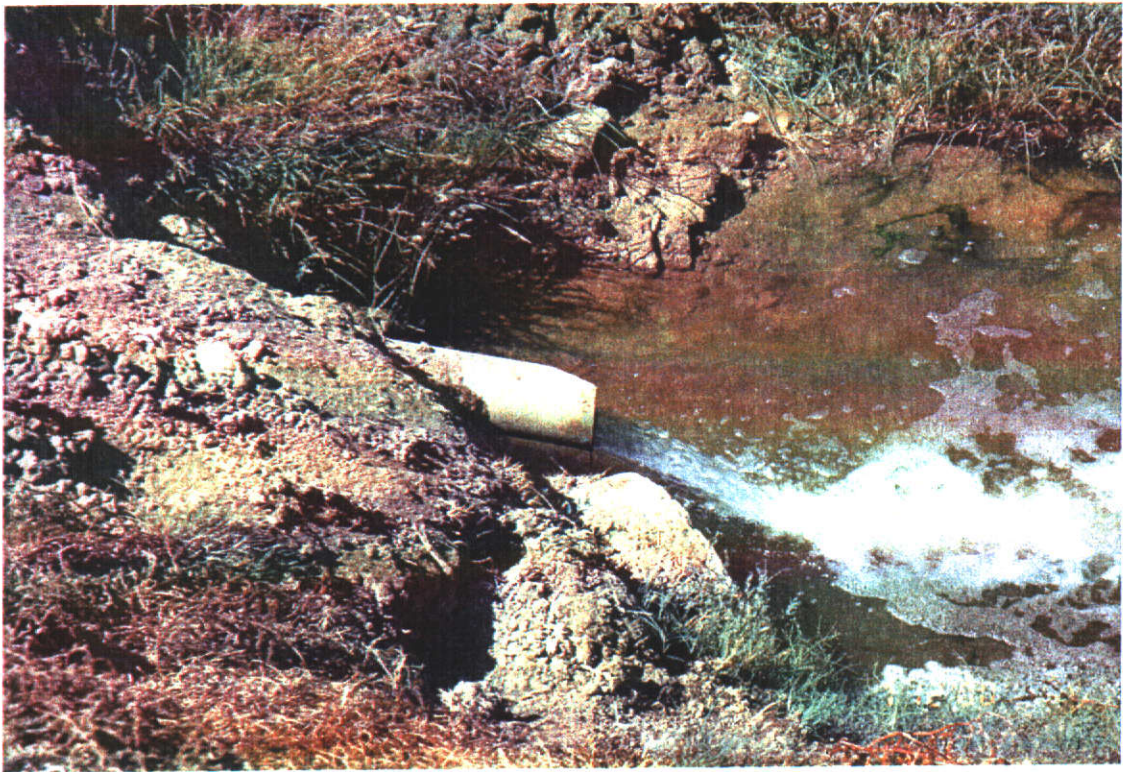
No. 13 Tile water discharging into main drainage ditch.
