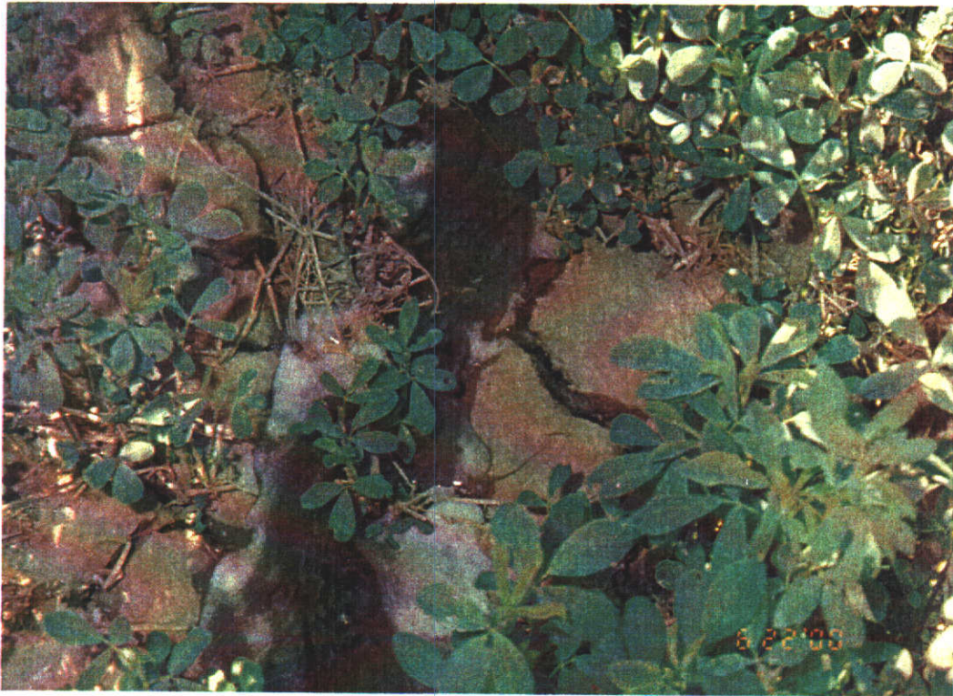
No.4 Water filling up cracks during an irrigation.
