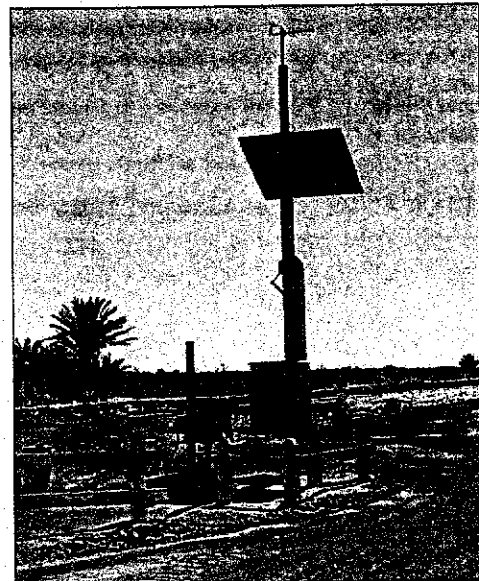
Solar Powered SCADA System
