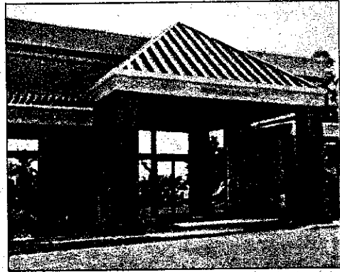
Water Control Center Entrance
