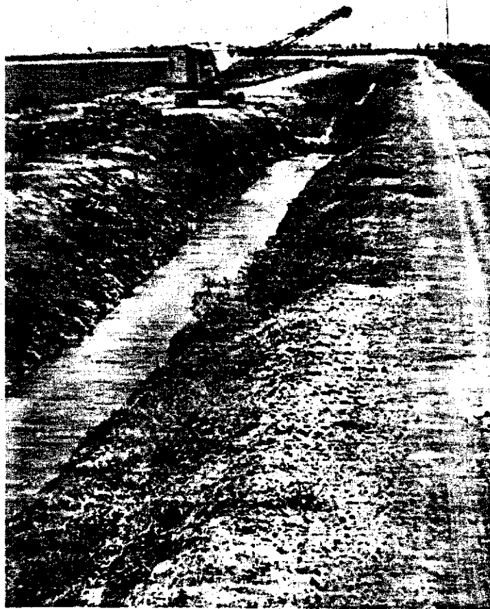
A DISTRICT DRAIN BEING CLEANED.
