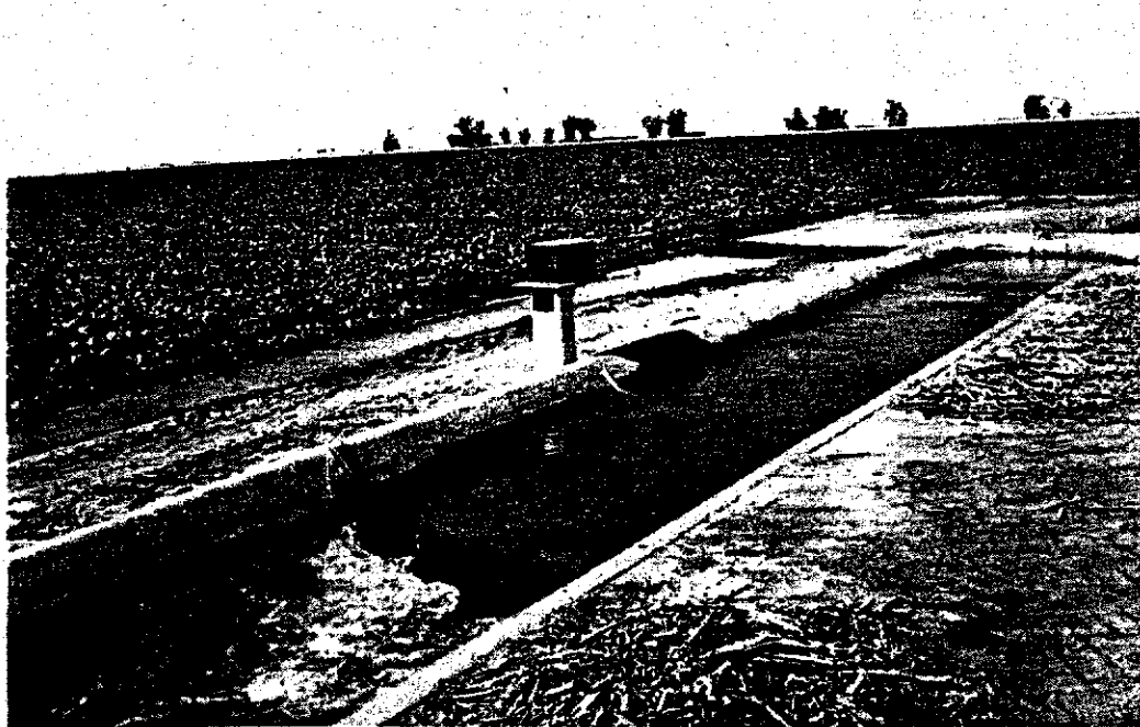
A WATER-LEVEL RECORDER IS RECORDING THE DELIVERY OVER A BROAD-CRESTED WEIR.
