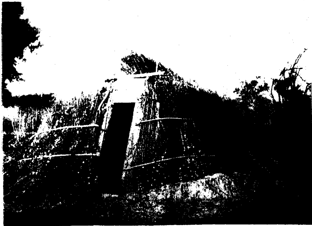
Figure 9. Chemehueve pit house showing method of anchoring structure with soil (Edward Curtis 1908).
