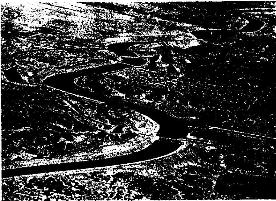
Gravity-flow 80-mile-long All-American Canal passes through mountains, sand dunes and raw desert en route from the Colorado River to Imperial Valley.
