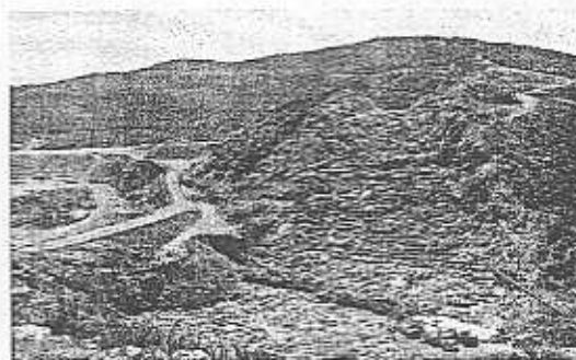
The Olivenhain Dam foundation exposes granodiorite rock that will support the future dam.
