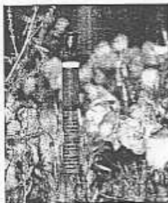
Purple fixtures are installed throughout the county where recycled water is used for irrigation.
