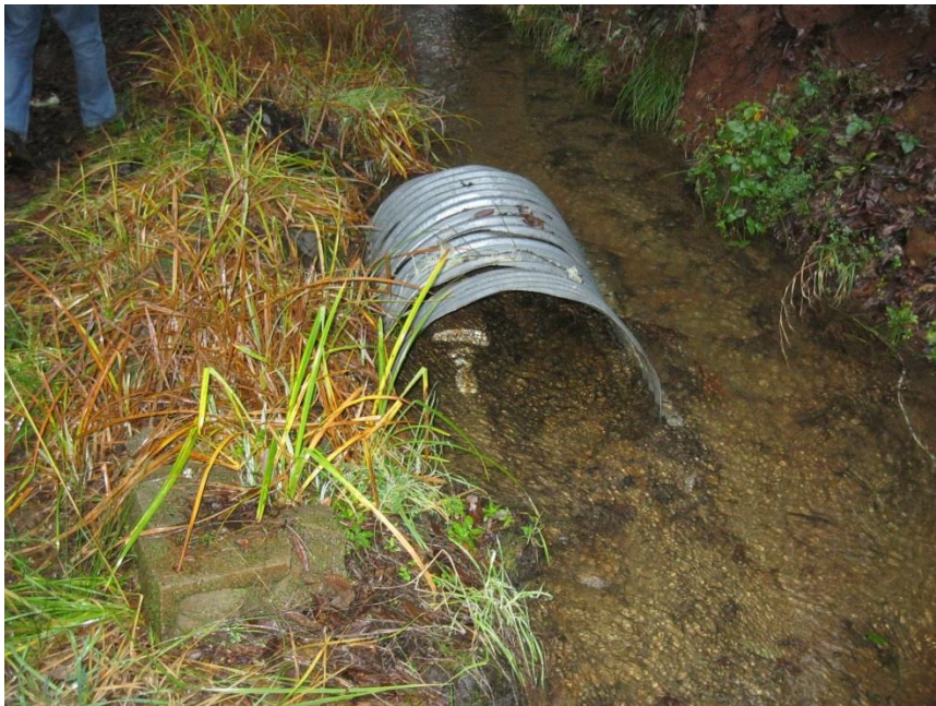
Photo 12 – Intake for water treatment facility.
