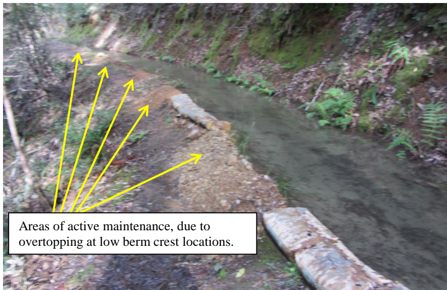
Photo 10 – limited free board space within the ditch.
