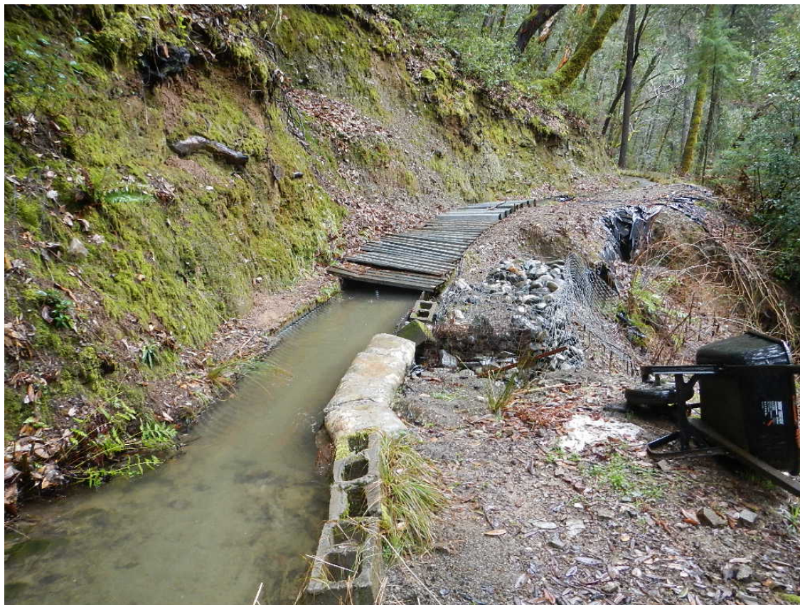
Figure 5. Repaired section of MMR ditch.
