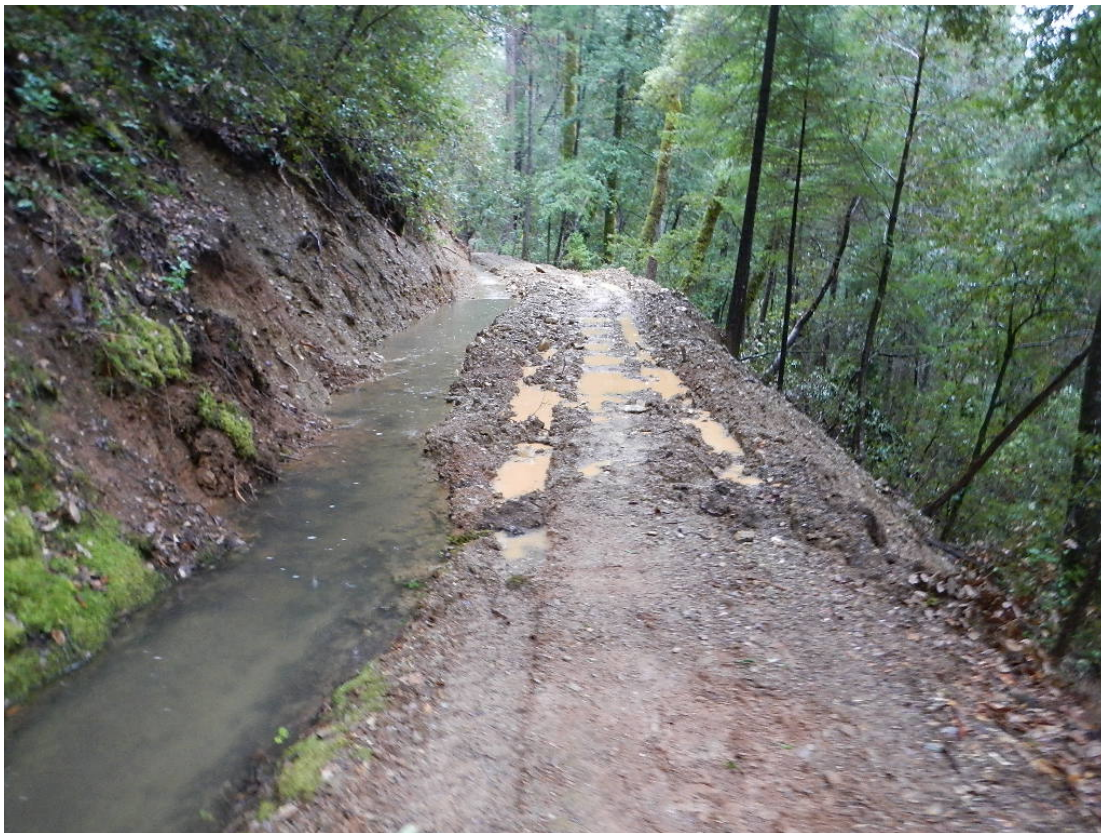
Figure 4. Recent MMR ditch repair site.
