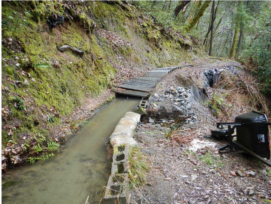
Figure 5. Repaired section of MMR ditch.
