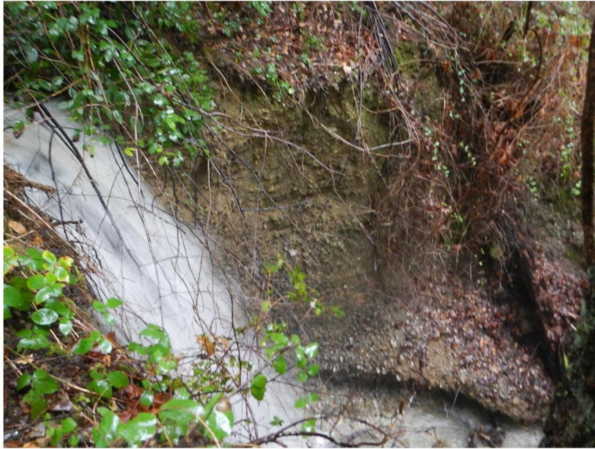
Figure 9. Gully headcut (approx. 15 feet deep) where MMR ditch leaves MMR into Irving Creek drainage.
