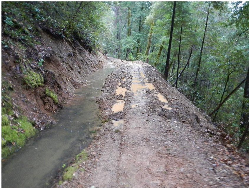
Figure 4. Recent MMR ditch repair site.
