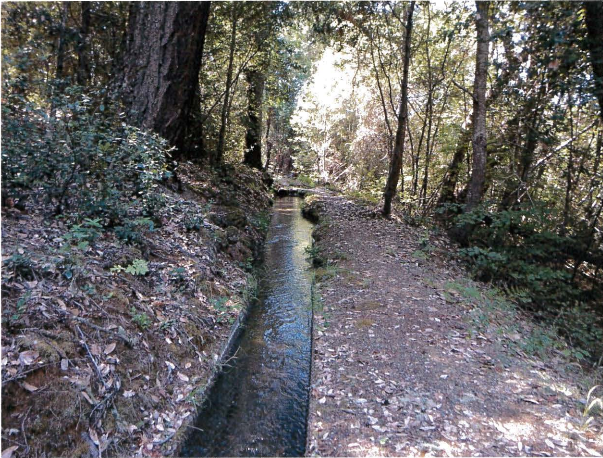
Photograph 9. HDPE pipe lining ditch.
