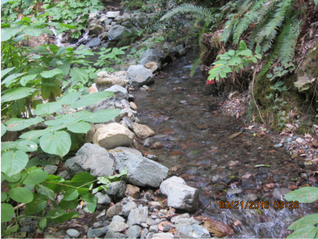
Exhibit MMR-02, Photograph #4 showing a portion of the diversion on September 21, 2016
