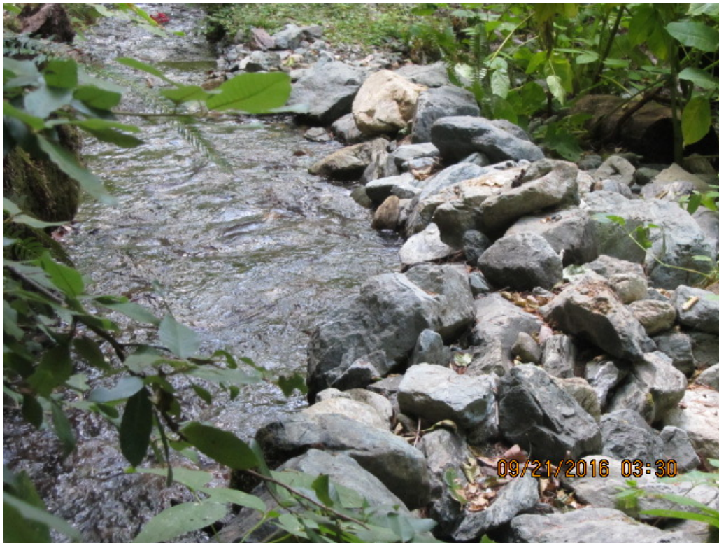
Exhibit MMR-02, Photograph #3 showing a portion of the diversion on September 21, 2016
