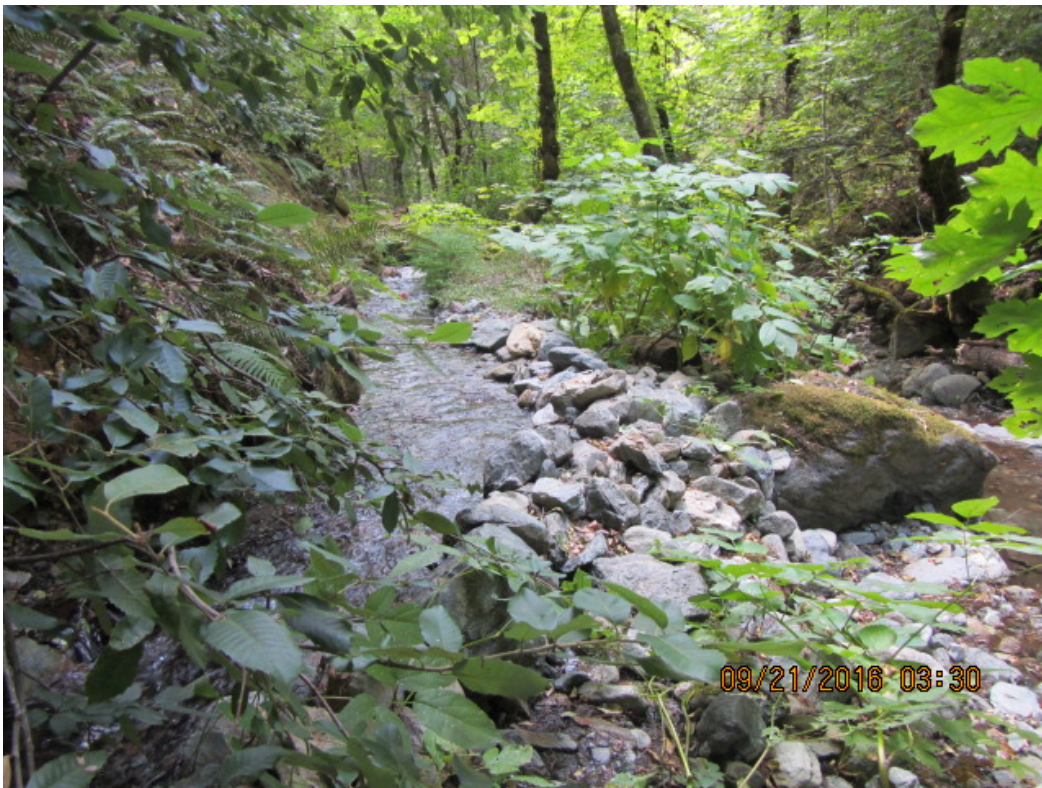
Exhibit MMR-02, Photograph #5 showing a portion of the diversion on September 21, 2016
