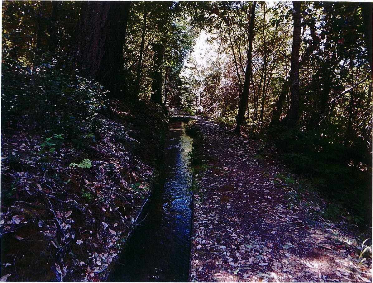
Photograph 9. HDPE pipe lining ditch.
