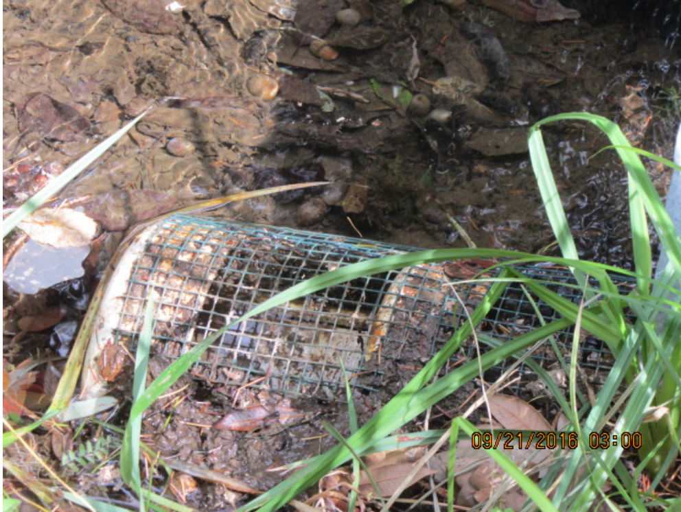
Exhibit MMR-08 Photograph #3 – A screen within the diversion hat is regularly cleaned and cleared of debris
