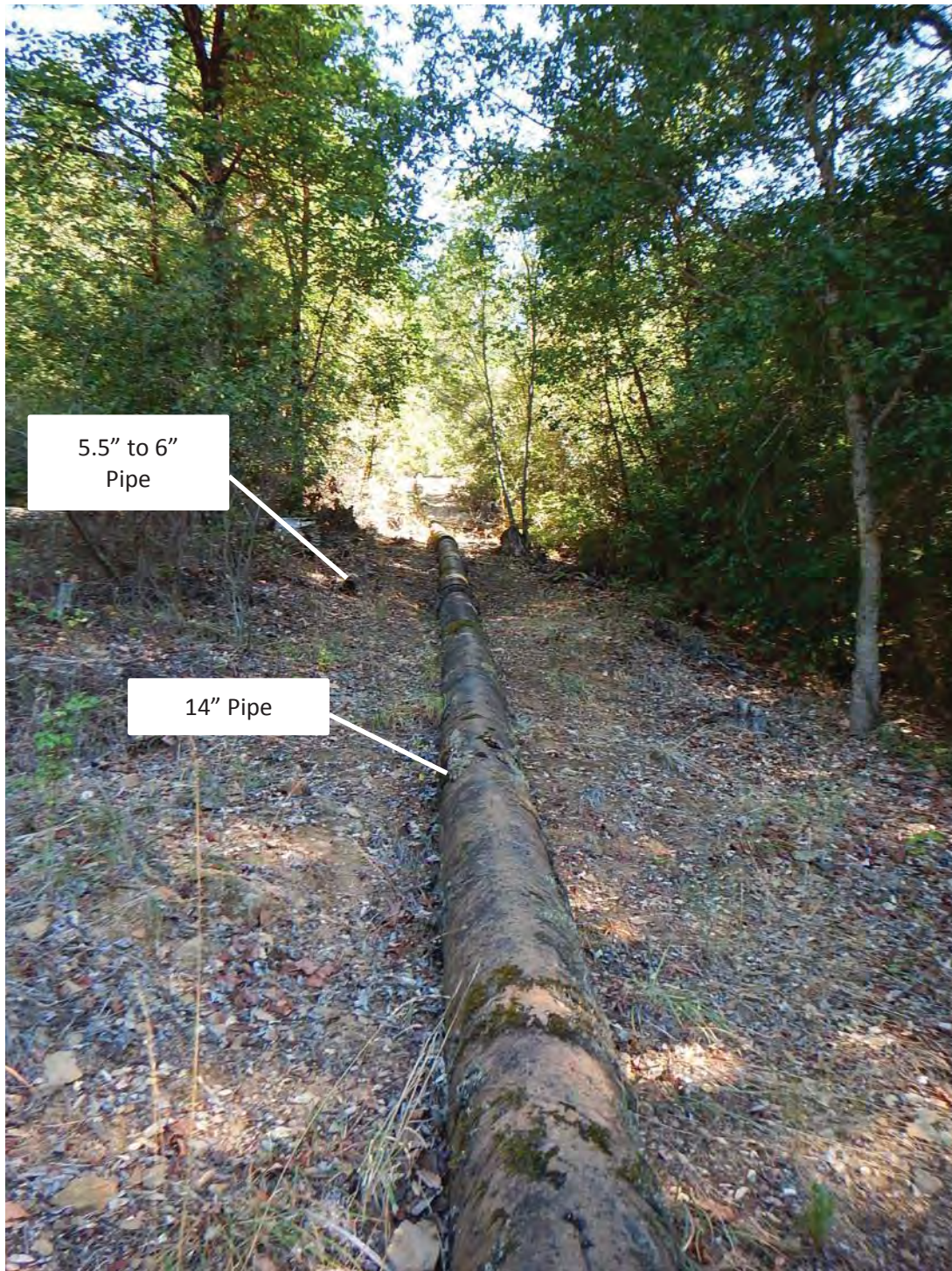
Photograph 2. 14" Diameter Penstock installed by Lue Hayes after he purchased the property in 1955.
