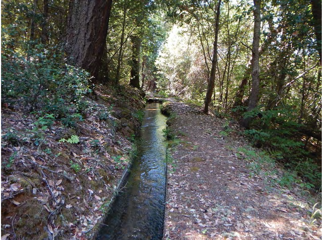
Photograph 9. HDPE pipe lining ditch.
