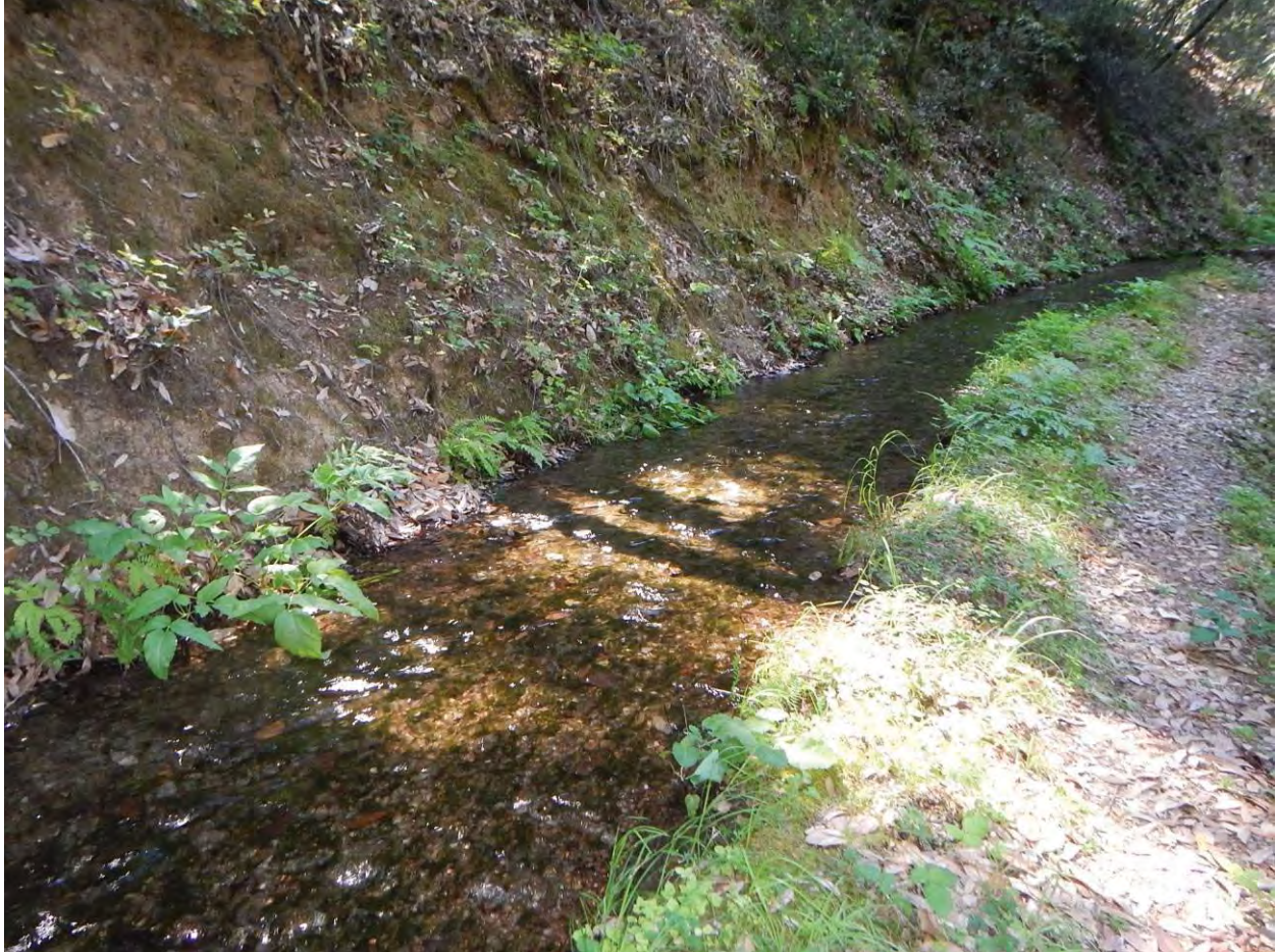
Photograph 10. Unlined ditch.
