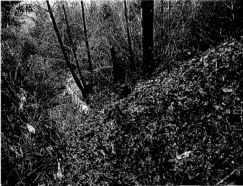
Photo 16 – 14-inch diameter penstock pipe.
