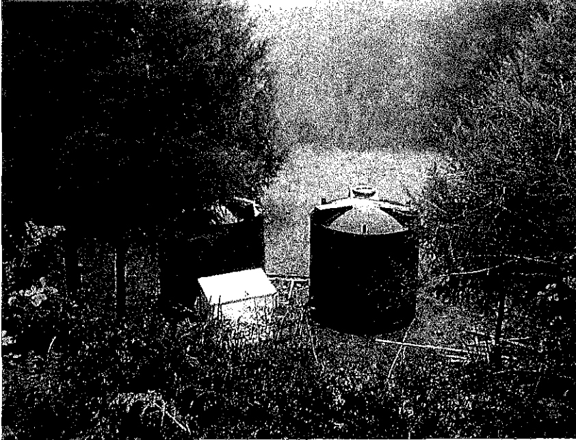
Photo 15 – (2) 3,000 gallon storage tanks.
