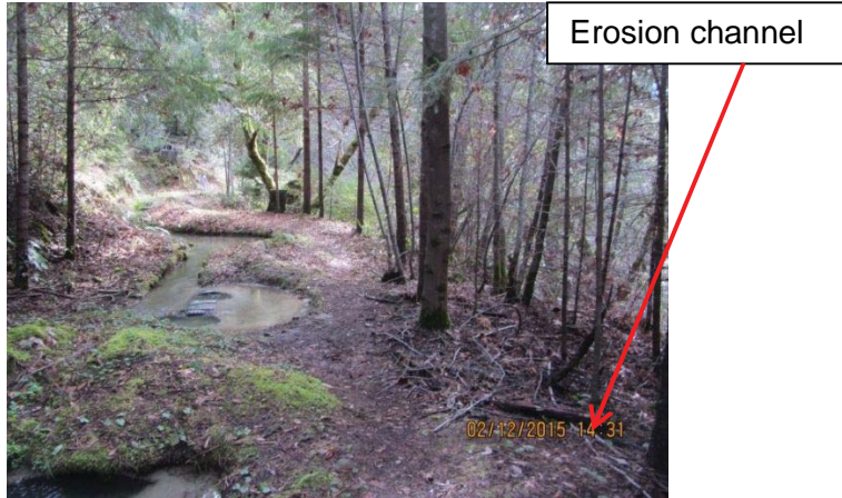
Image 5- shows Point 3, a tank or railroad tank car buried in the ditch channel, likely intended to trap sediment. The tank car is full of sediment. Water flowing in the ditch appears to have overtopped the outboard berm at this location and caused some erosion on the slopes below. (Photo 8467)
