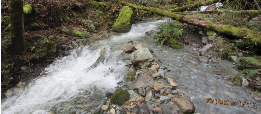
Image 3- shows Point 1, the Point of Diversion. The Stanshaw Diversion flows toward the lower right corner of this image. It appears the rock and cobble diversion structure fails episodically and likely requires periodic modification as Stanshaw Creek's flows change, in order to maintain a diverted flow. (Photos 8459, 8460 and 8461 stitched)
