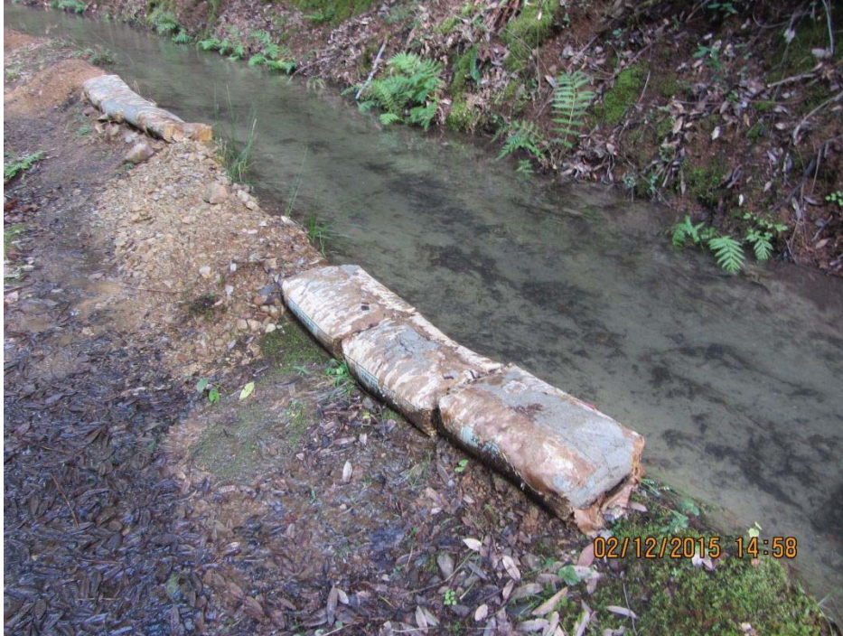
Image 19- Point 12, closer view of berm repair made with ready crete concrete sacks and soils. Note the saturated soils along the outboard berm where water is seeping. (Photo 8510)
