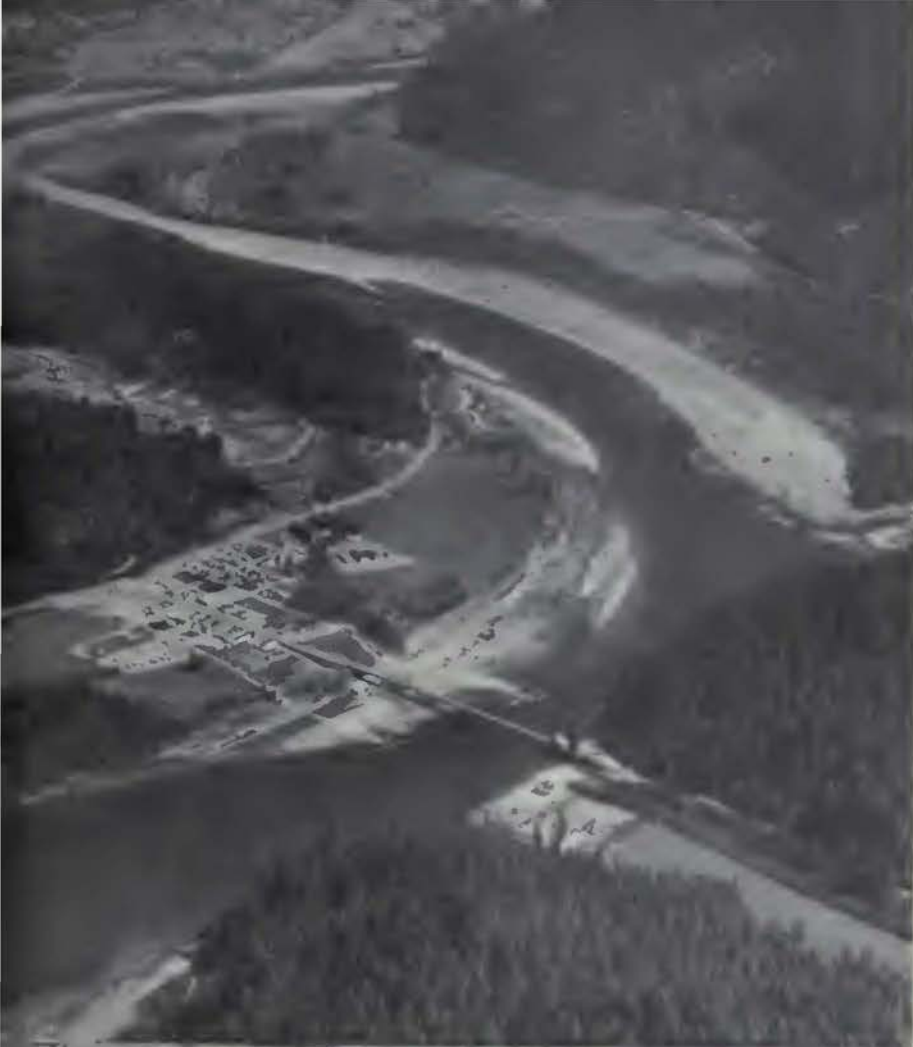
Below: Town of Klamath December 1955
