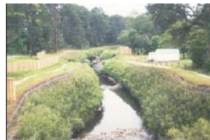
Figure 7.33 Established VRSS Structure (Sotir and Fischenich, 2003)
