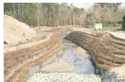
Figure 7.32 VRSS Structure After Construction (Sotir and Fischenich, 2003)
