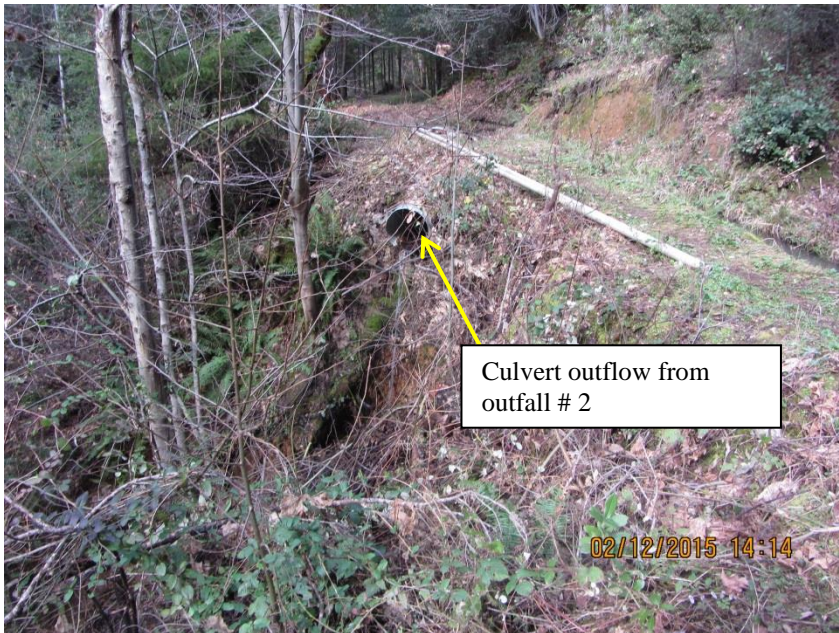
Photo 6 – This photo shows the outflow from Outfall # 2 on the diversion ditch.
