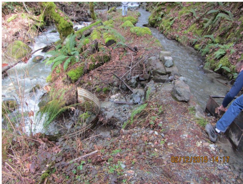
Photo 4 – Outfall structure located 50-feet downstream of POD.
