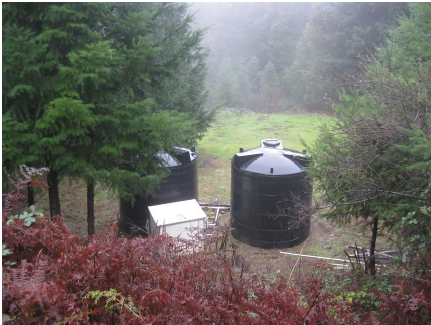
Photo 15 – (2) 3,000 gallon storage tanks.
