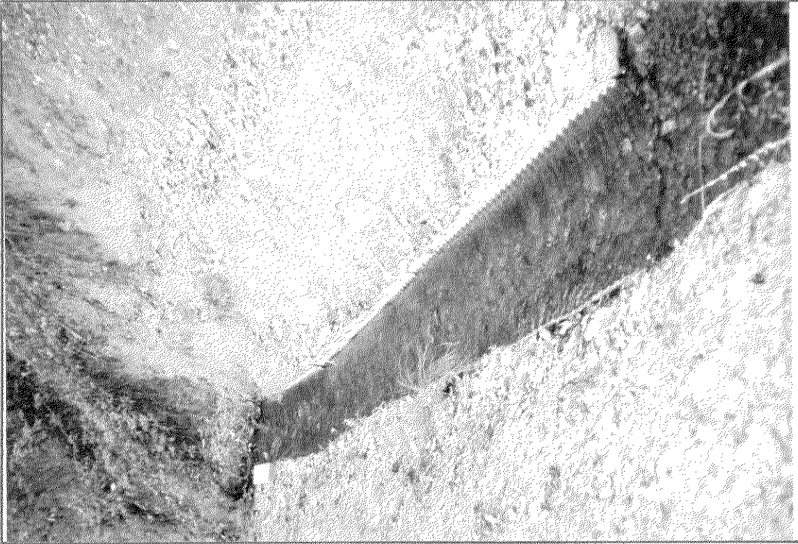
Photo 20. Half-culvert in ditch.
