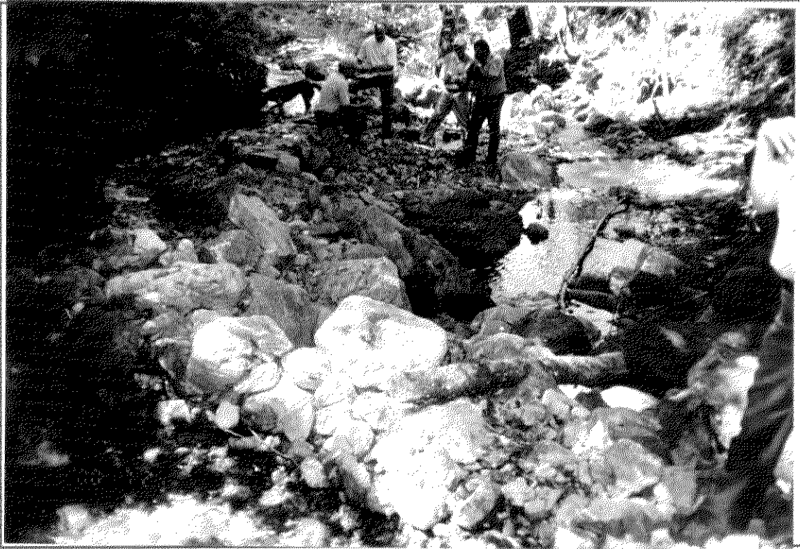
Photo 15. The POD looking downstream. The diversion ditch is on the left. Note the “diversion rocks” in foreground.
