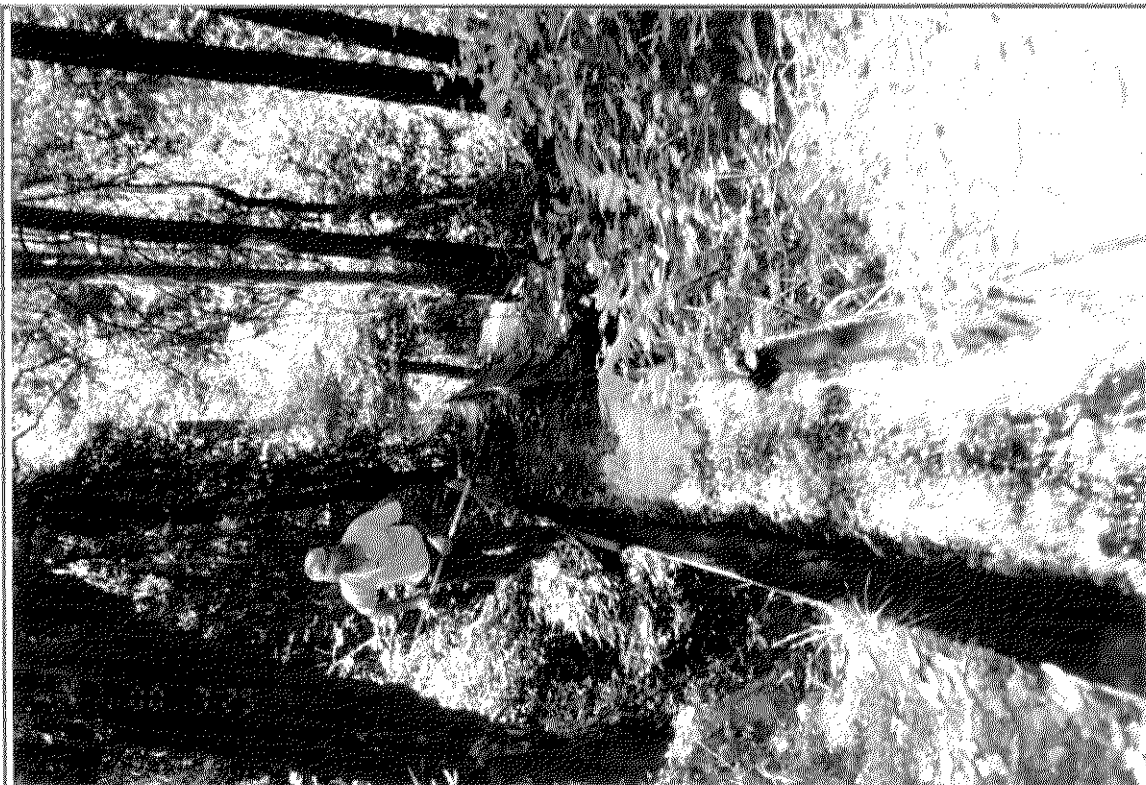
Photo 25. Mr. Cole clearing the trash rack of leaf litter. Clearing is done daily and > 5 times per day during the fall. Water then enters a holding tank, thence penstock.
