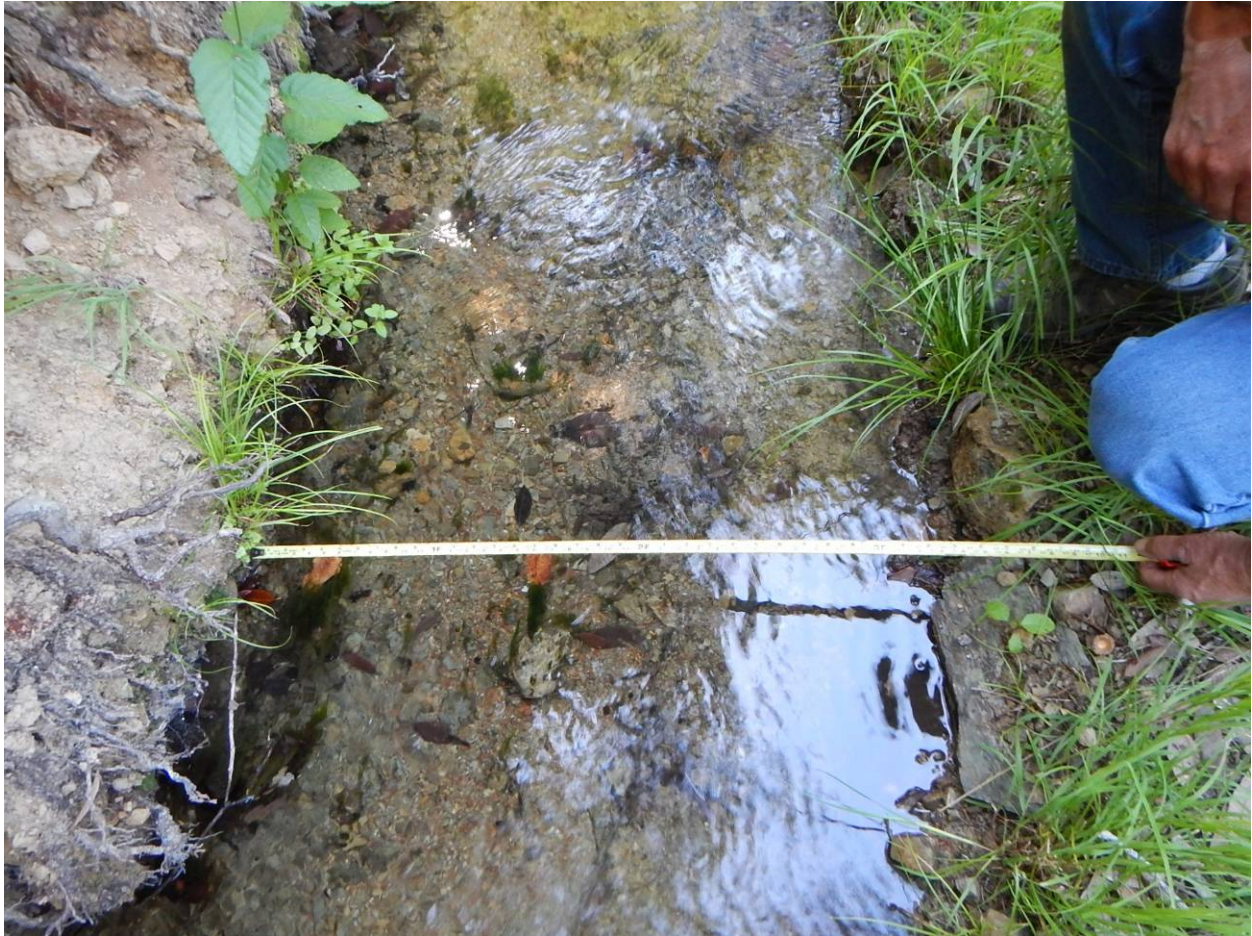
Photograph 11. Narrow location in canal, top width about 3.3 feet
