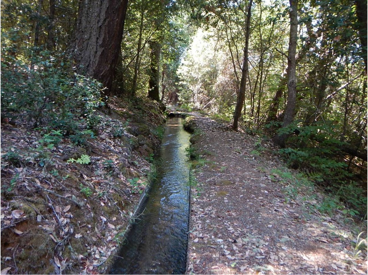
Photograph 9. HDPE pipe lining ditch.
