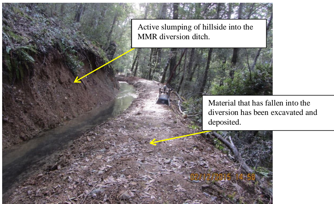
Photo 9 – Area of active slumping into MMR Diversion ditch.
