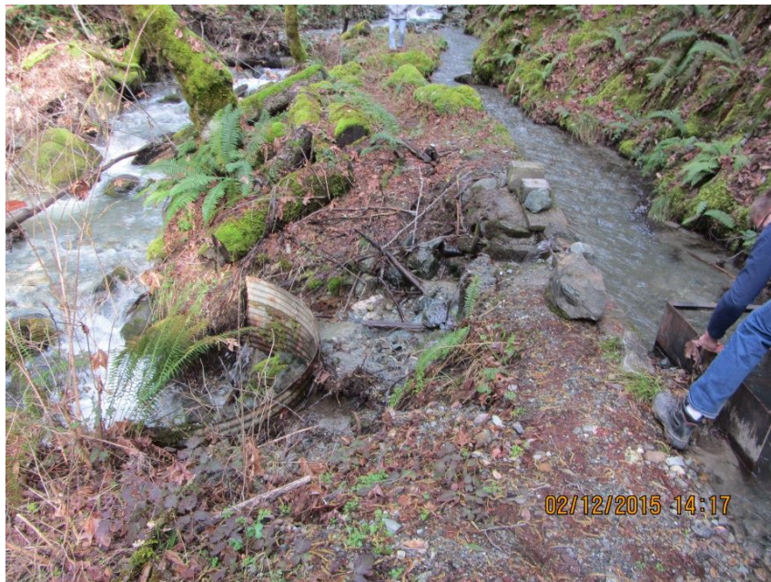
Photo 4 – Outfall structure located 50-feet downstream of POD.
