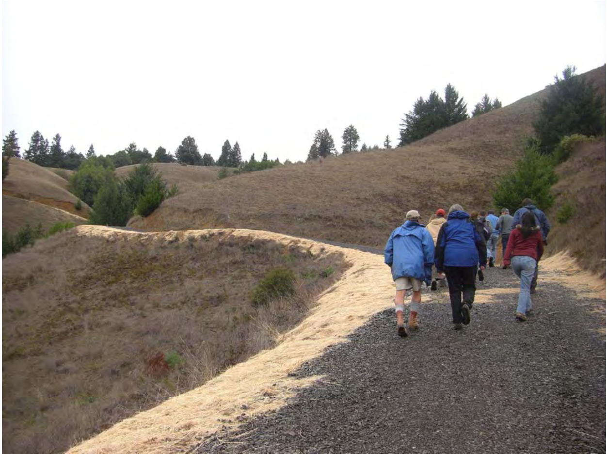
Figure 17: This road was changed from insloped to outsloped as a Fish Friendly Farming project to reduce fine sediment generation and delivery.
