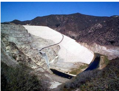
The U.S. Army Corps of Engineers concluded that the use of Seven Oaks Dam, pictured here from upstream, for conservation storage is feasible, beneficial, and compatible with the dam's flood-control functions.
