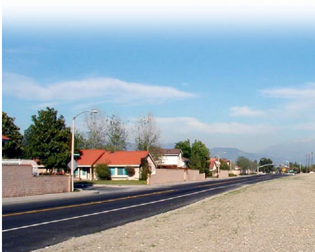
Some pipeline construction will be in established rights-of-way. Construction will temporarily disrupt some portions of roadways, possibly requiring the temporary use of alternate routes.
