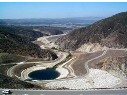
Looking southwest from the crest of Seven Oaks Dam, the plunge pool, pictured here in the foreground, with the Santa Ana River in the background, is in an area that was periodically inundated when floods occurred. The Seven Oaks Dam has dramatically reduced the potential for flooding downstream from this area.
