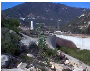
Devil Canyon Power Plant of the State Water Project.
