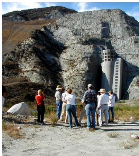
The U.S. Army Corps of Engineers would be requested to approve alterations to the Seven Oaks Dam, including proposed changes to the intake structure pictured here.
