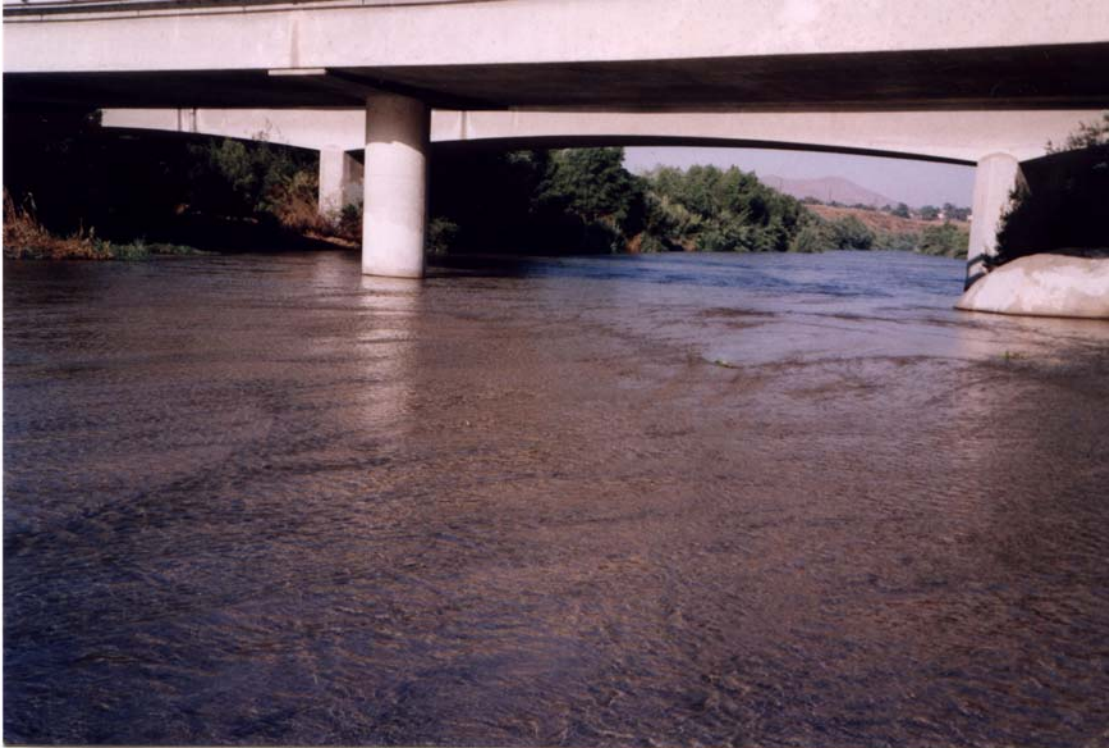
Photo 8. The Santa Ana River at the Van Buren Street bridge.
