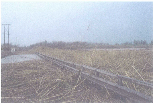
River Road Bridge in the 2005 Floods
