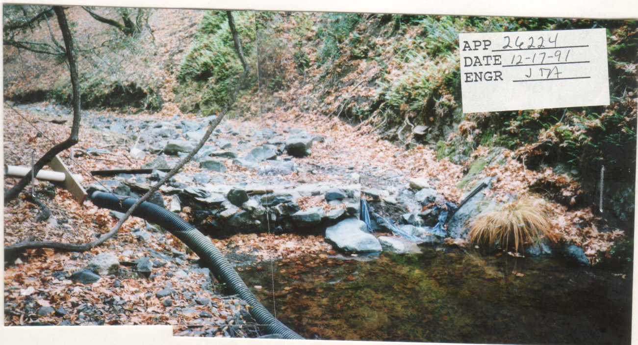
Picture during revisit - Structure has been removed In Order To Recut To Conform to By-Pass Requirements
