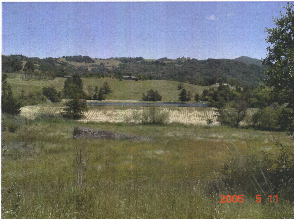
Overall view of the reservoir looking north east from River Road.
