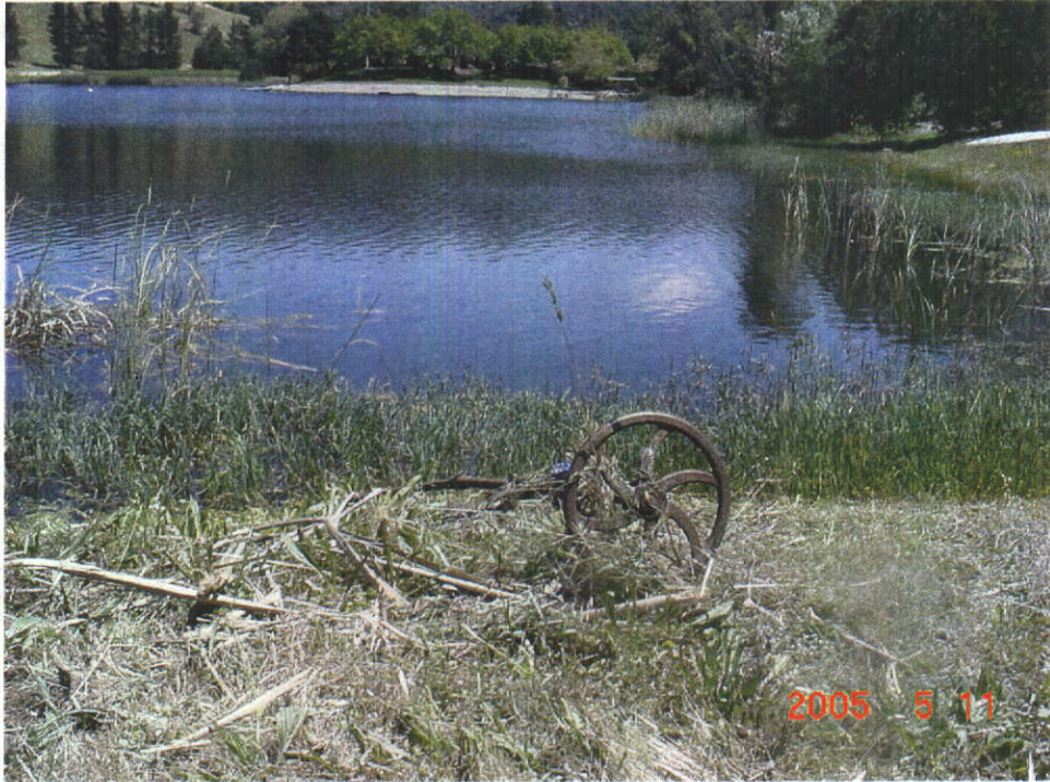
Outlet valve control handle at south west corner of lake.
