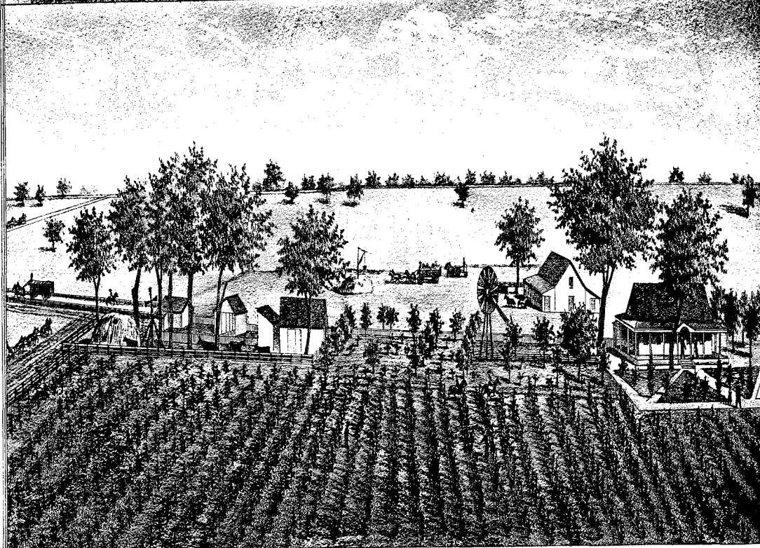
RES. 388 RANCH OF ALDEN HAMMOND, ONE 1/2 MI. SAN JOAQUIN COUNTY, CALIFORNIA.
