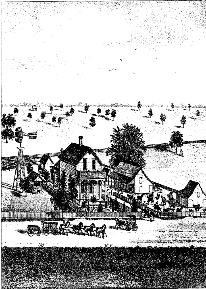
RESIDENCE OF U. J. MUNSON, ATLANTA, SAN JOAQUIN CO CAL.
