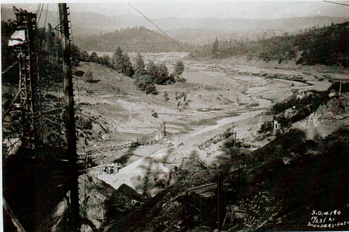
Figure 2. Historical photo of Gravelly Valley during the construction of Scott Dam. Trees from the flood plain have been logged in anticipation of reservoir filling. Photo from the Heald-Poage Museum in Ukiah, CA.
