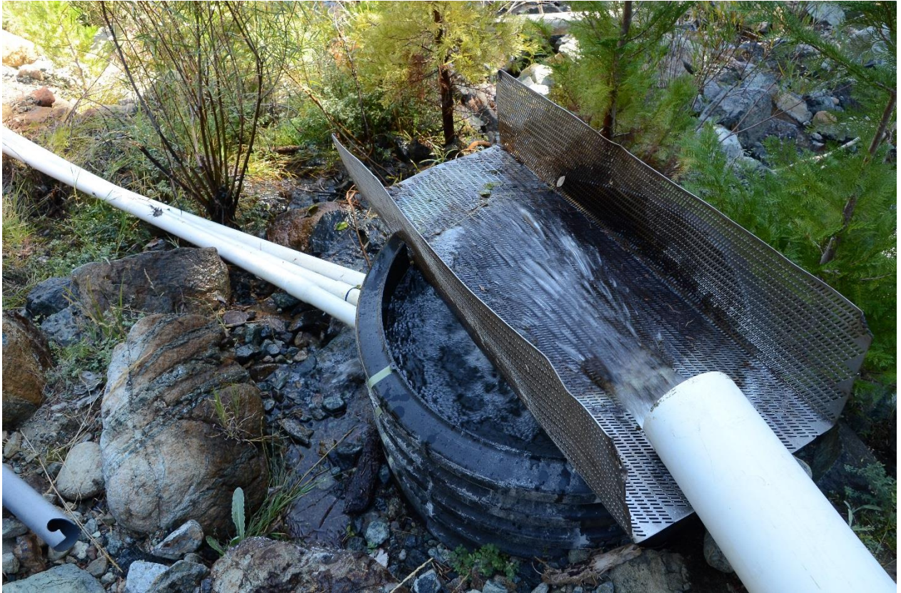
Figure 2. A single diversion pipe feeds a spring box where three separate pipes convey diverted water for power supply and irrigation.
