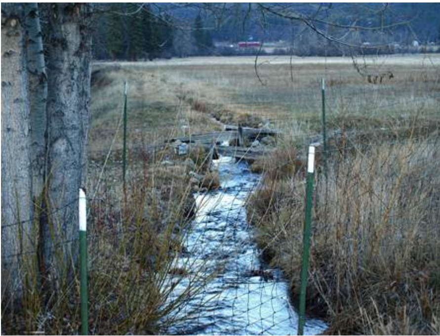
Ditch from Shakleford Creek running full in December 2009
