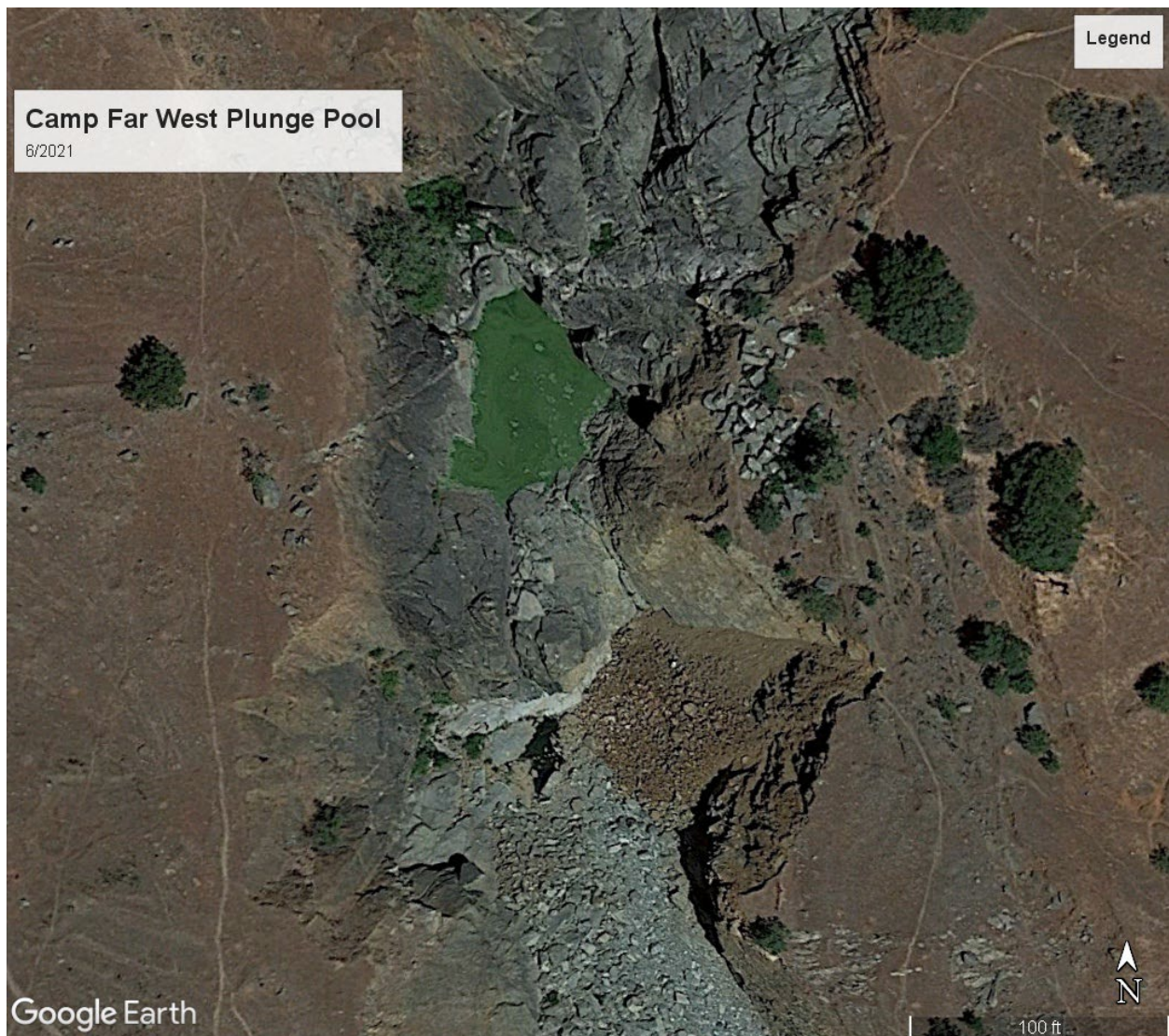
Figure A3. June 3, 2021 Google Earth aerial image of Camp Far West spillway plunge pool
