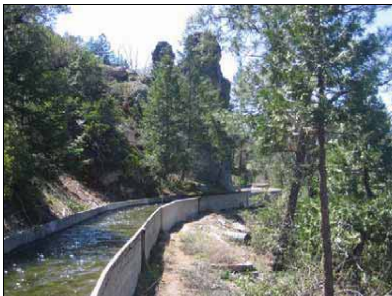
Feature 3: Concrete Canal. Facing: West (Photo acc. # 482-12-2-52)
