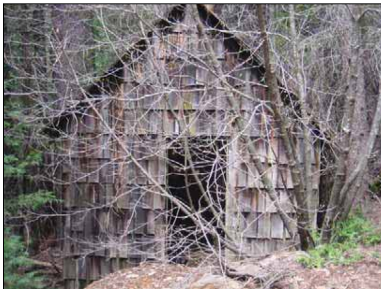
Feature 5: "Kilarc Shack 2" Ditch Tender Cabin. Facing: Northeast (Photo acc. # 482-12-1-60)
