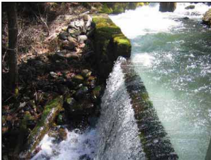
Feature 2: Diversion Dam. Facing: Northeast (Photo acc. # 482-12-1-39)
